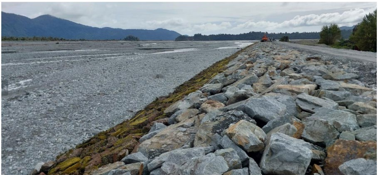
Figure 10: contractors placing rock-armour full batter on the Havill wall stopbank
