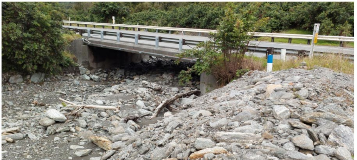
Figure 13: View of Stony Creek at SH6 bridge looking upstream
