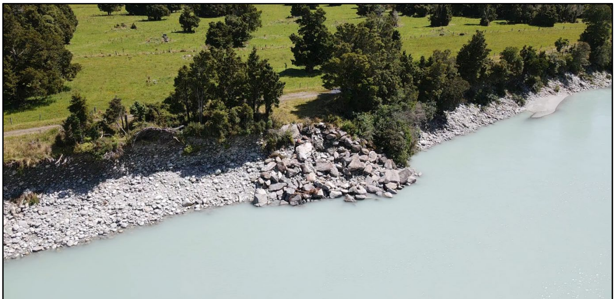
Figure 7: Spur 3 requiring remediation
