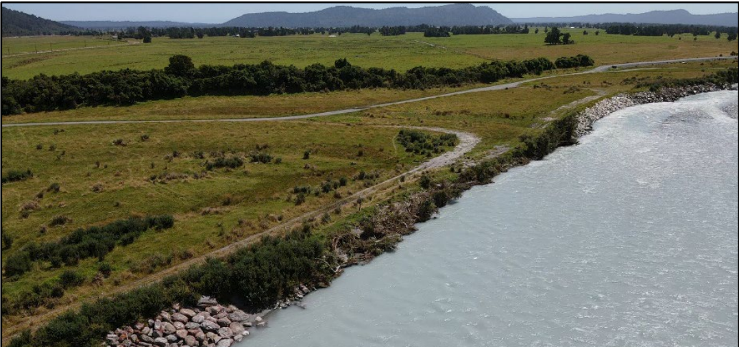
Figure 1: Wanganui downstream of SH6 pre works.
