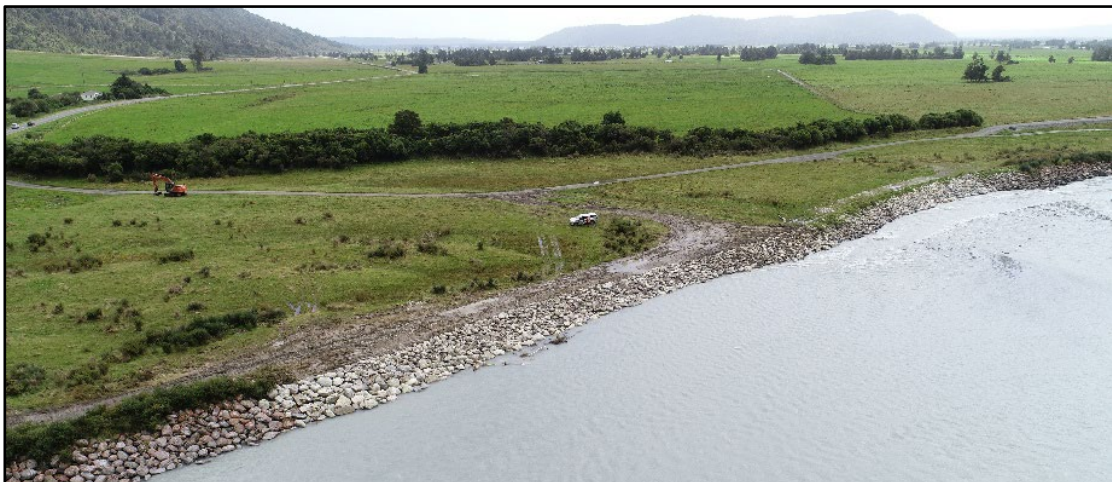
Figure 3: Wanganui downstream of SH6 - post works
