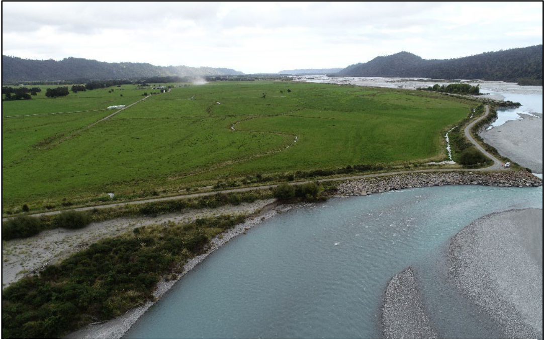
Figure 4: Blackburn's - pre works
