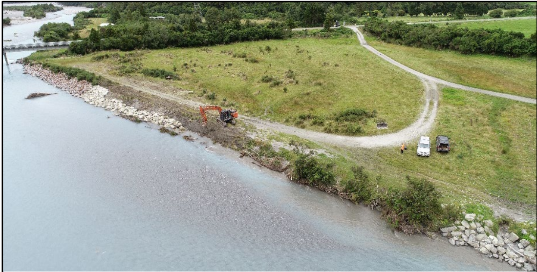
Figure 2: Wanganui downstream of SH6 - during works
