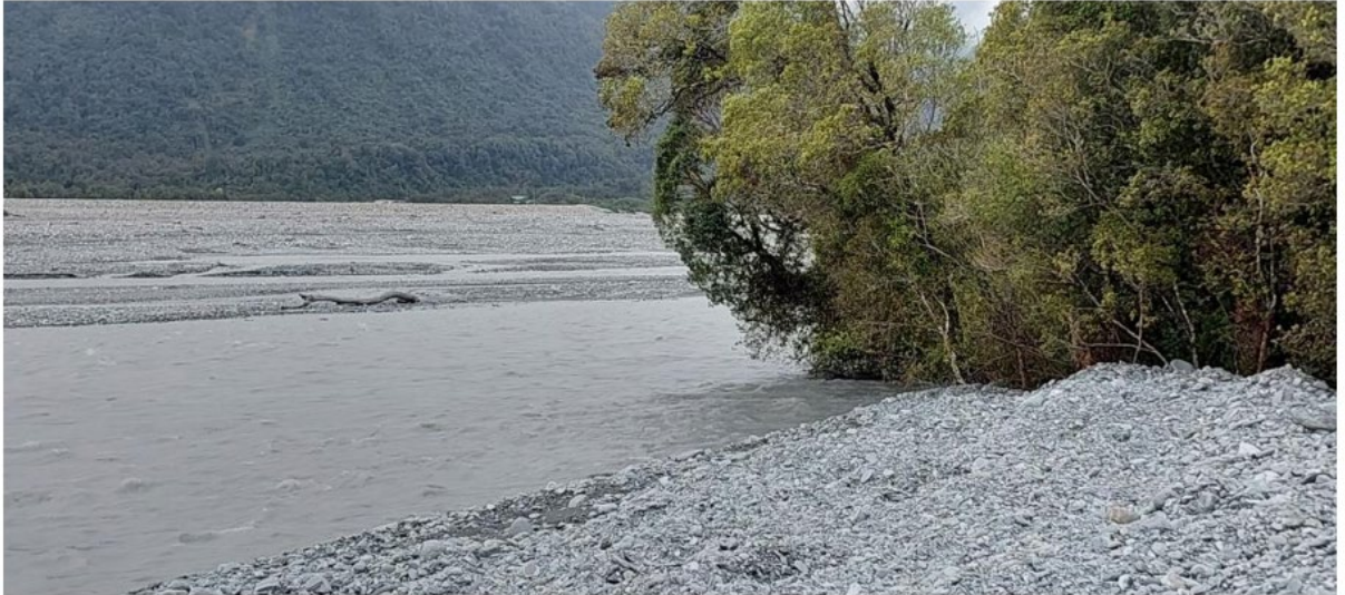
Figure 11: Flow within multiple braids at Canavan's Knob (trees) looking upstream standing on the river training bund.
