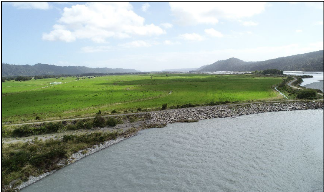
Figure 5: Blackburn's - post works
